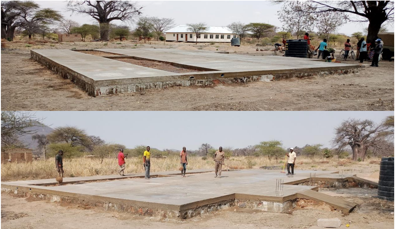
Photo #7: Completion of oversight concrete
