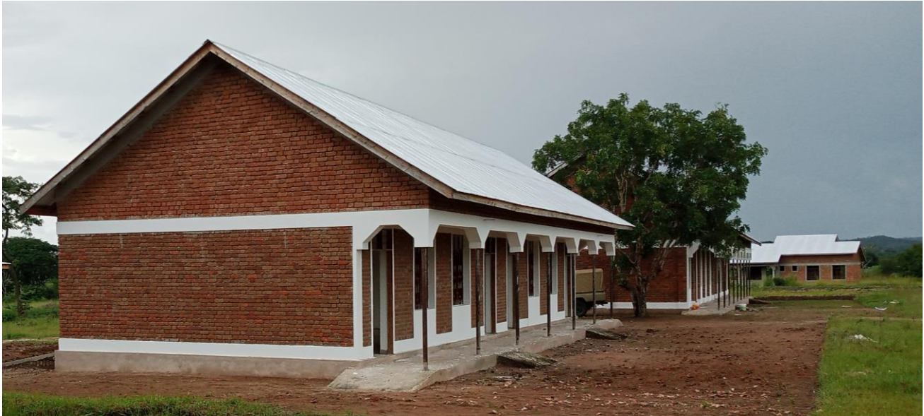
Photo # 3: As you can see in the picture above, the dormitory building is 100% complete.
