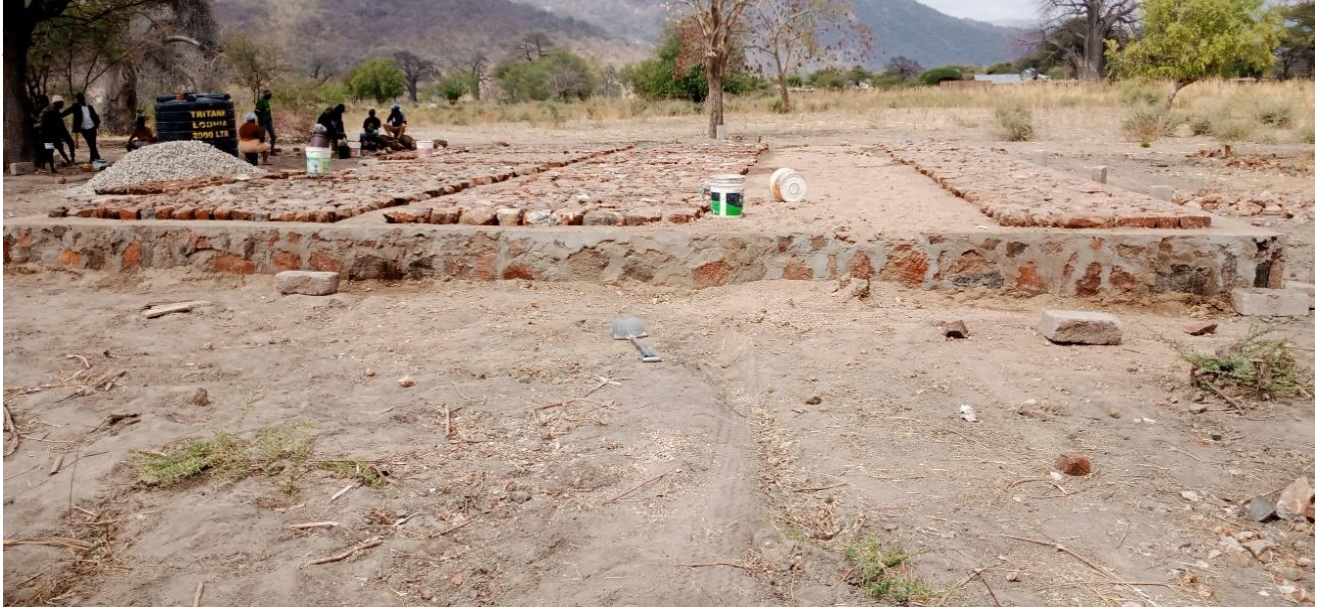
Photo #5 The completed hardcore foundation
