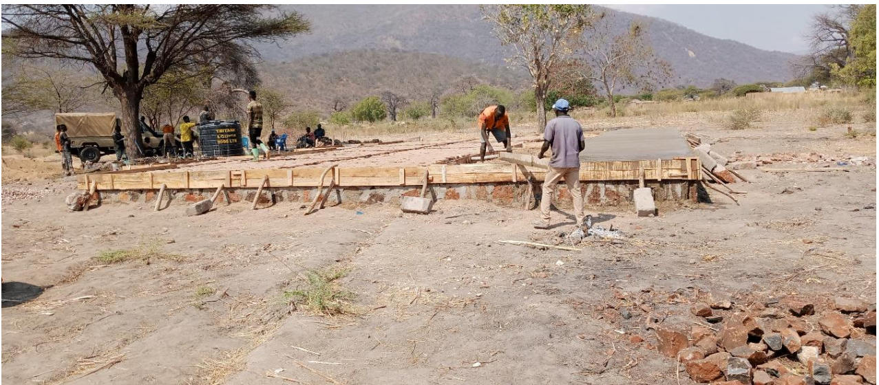
Photo #6: formwork and reinforcement bars around the foundation base
