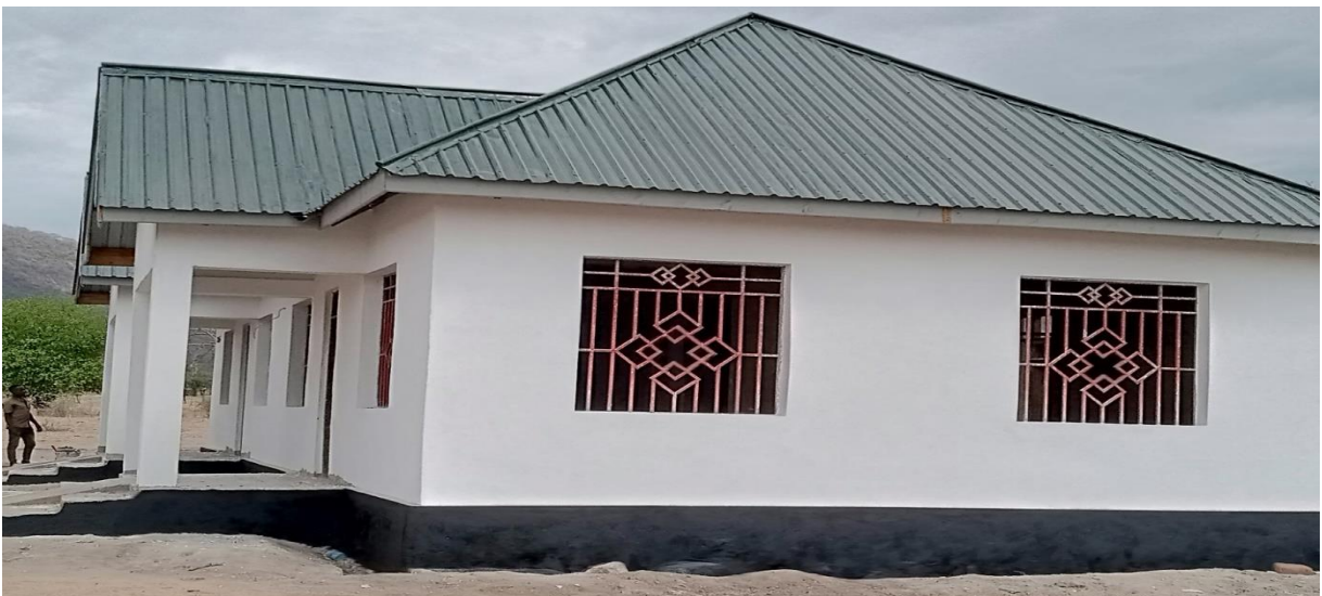
Photo # 12: Skimming internal and external walls
