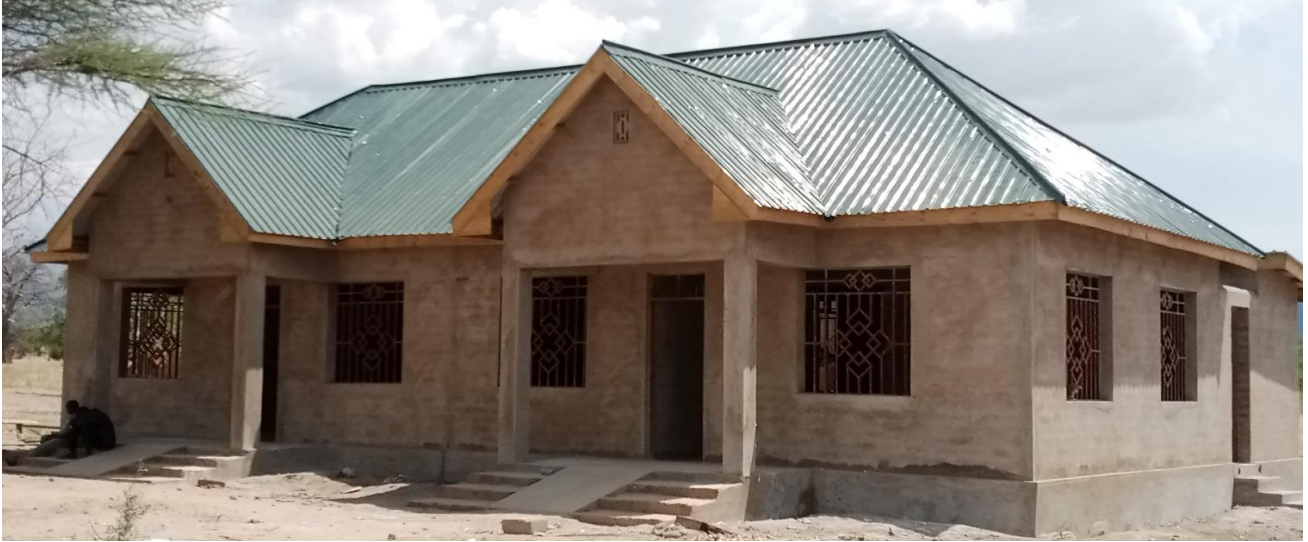
Photo #11: Plastering, window grill, and door frames
