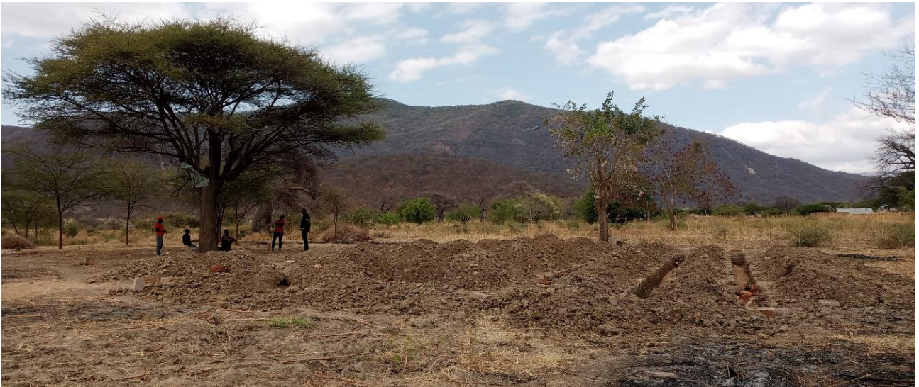
The foundation of the two-in-one house of health providers
