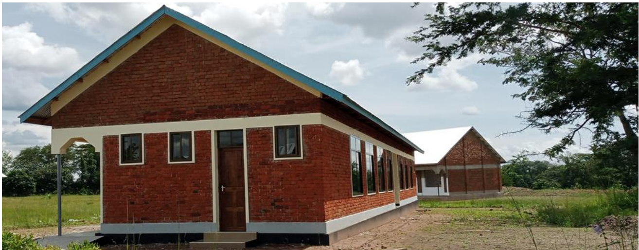
Photo # 3: Administration block side elevation
