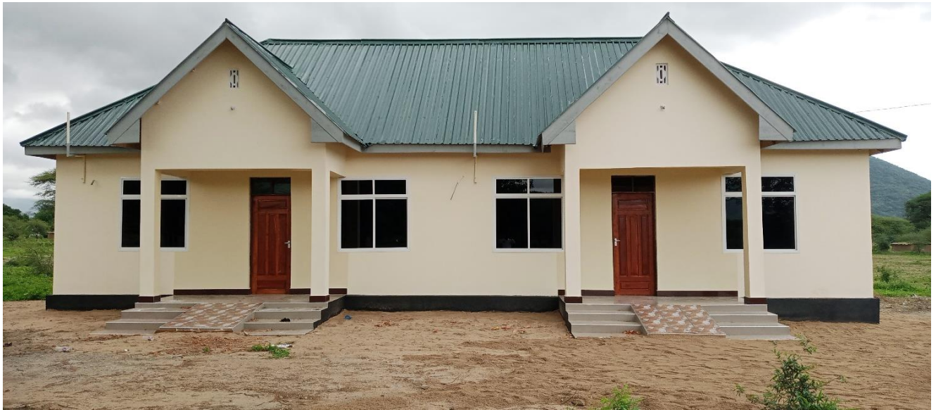
Photo #13: Completed two-in-one staff houses
