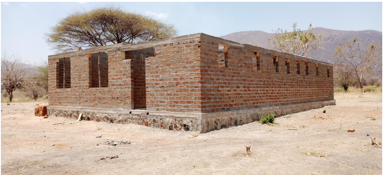
Photo #10: Shows the Ring beam
