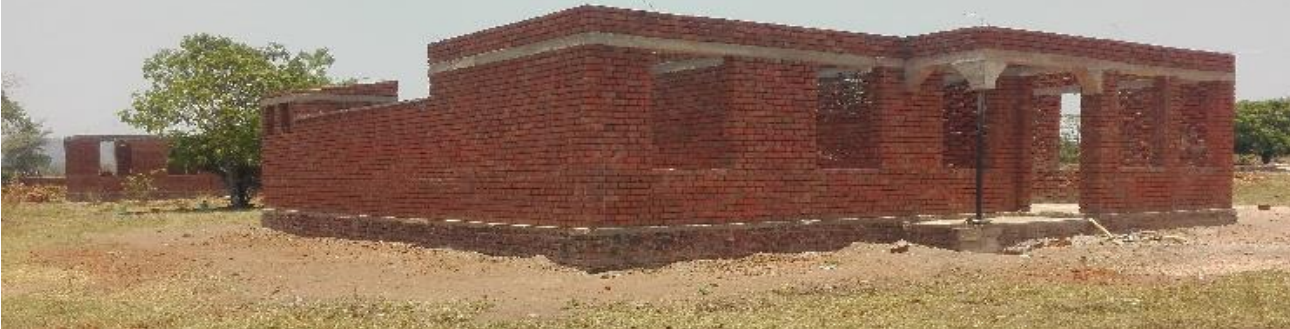
Photo # 11: wall construction independent house
