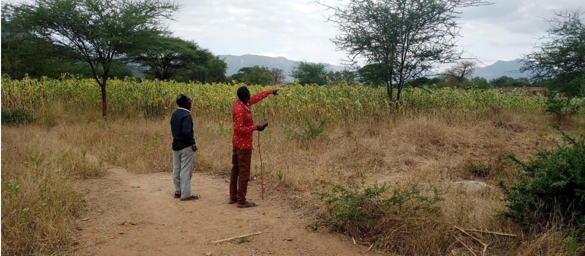
Photo #.....: Sub-Village Chairperson directing the construction site
