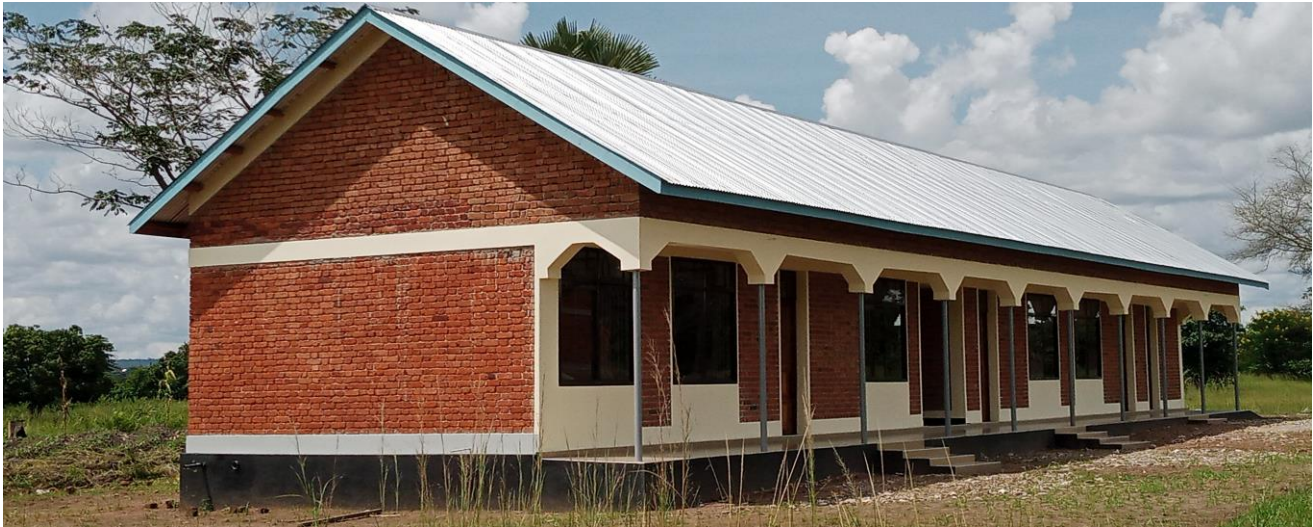
Photo # 2: Administration block front elevation
